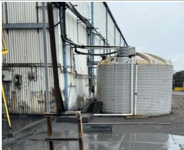
Photo 8 – Stormwater Storage Tanks
