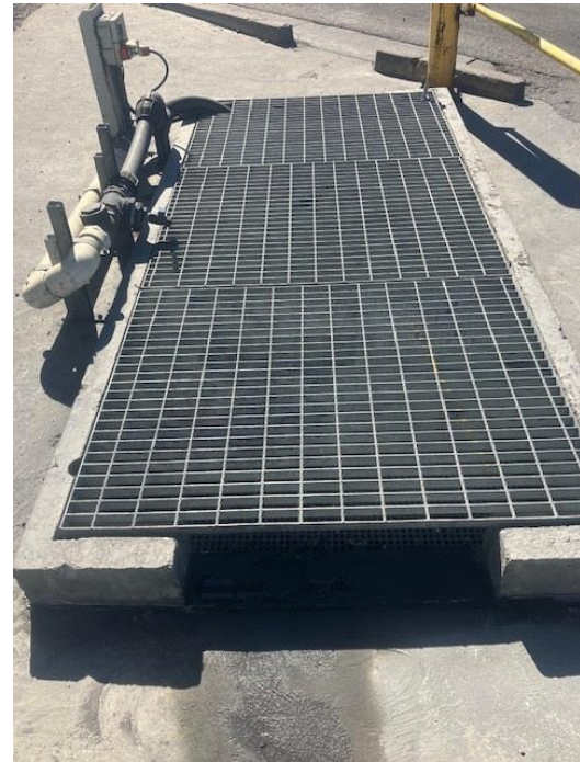
Photo 4 – Stormwater Interception Sump
